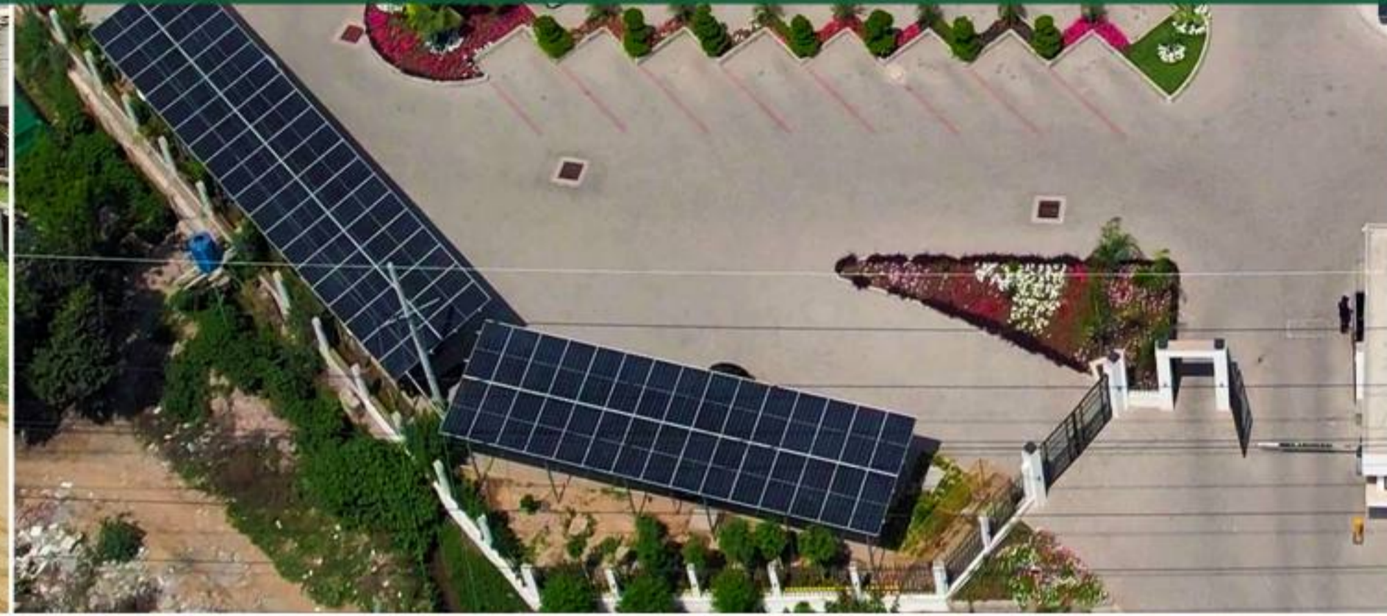
75 kW Solar Power Plant at Saleem Memorial Hospital, Lahore
